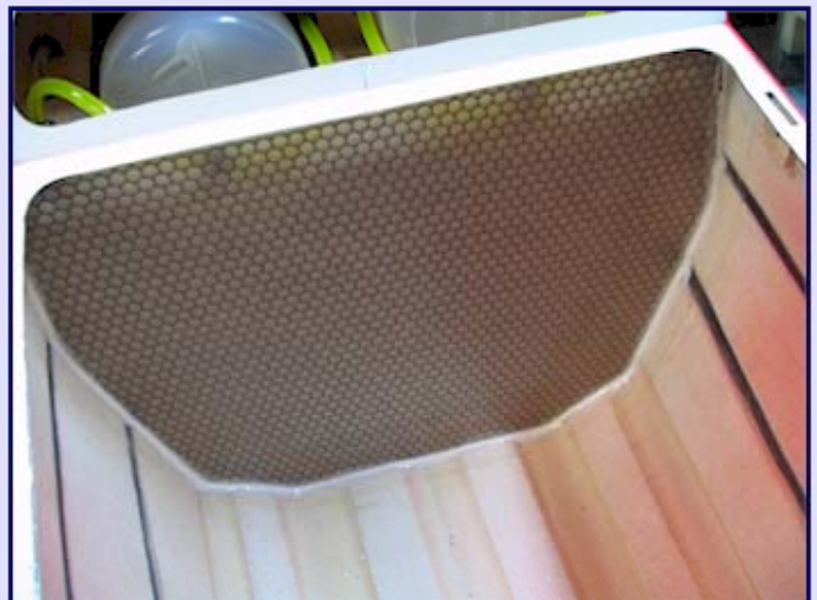
Honeycomb Bulkhead
